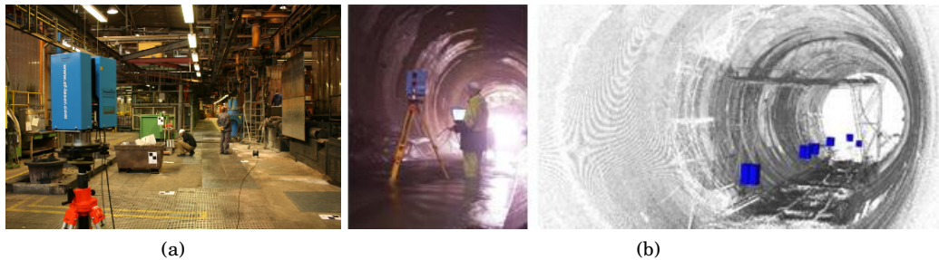
Fig. 1: A 360° laser scanner of inmetris3D placed in a production hall (a) and in a tunnel with the resulting scan data (b). (All images courtesy of inmetris3D.)
